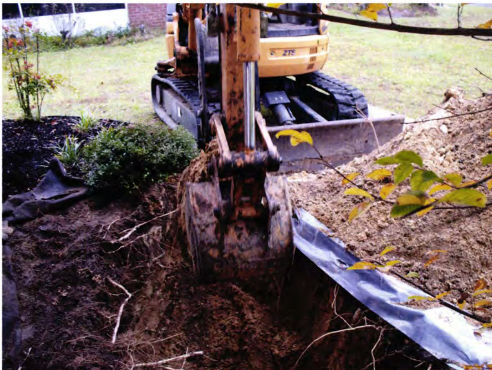
Picture 2: UST 538LaurelBB excavation in progress.
